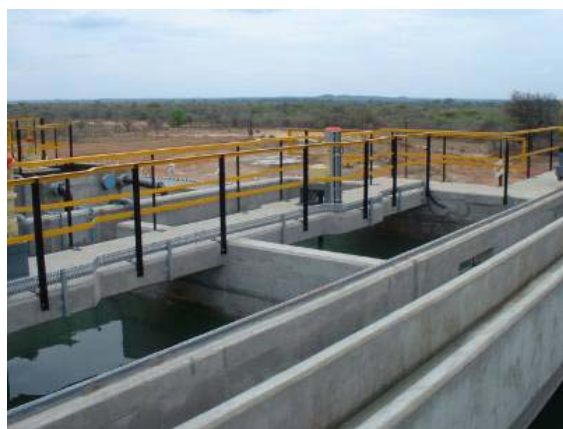
6. Complete-mix reactor for gypsum crystallization
