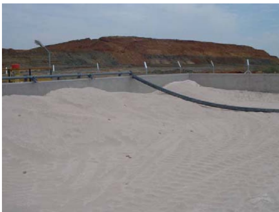
3. Limestone handling and dosing system.
